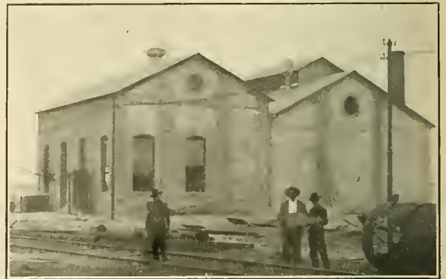
EXTERIOR VIEW OF POWER HOUSE, SHOWING CHARACTER OF CONCRETE BUILDING CONSTRUCTION.
